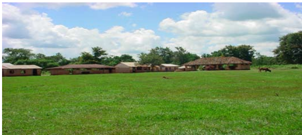
Figure 3: Dilapidated Structures at Naluwori Primary School in Butansi Subcounty
